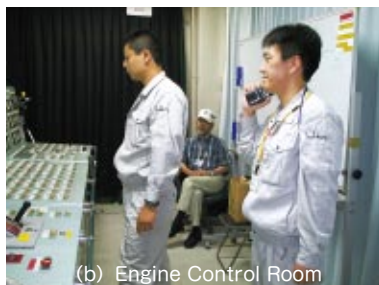
(b) Engine Control Room
